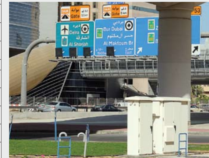
Scada System Cabinet at Shaikh Zayed Road, Dubai
